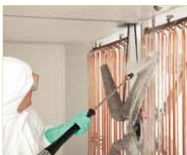
^ The S-line is easy to clean, even with high-pressure water equipment.
